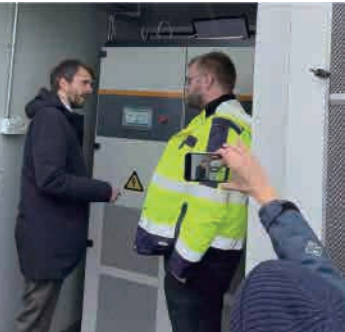
PV-ESS-EV Charging Station Project in Norway
